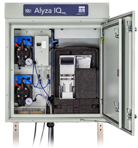
PARAMETER: Orthophosphate APPLICATION: Phosphate Dosing in Drinking Water INSTRUMENT: YSI Alyza PO 4 Orthophosphate Analyzer
